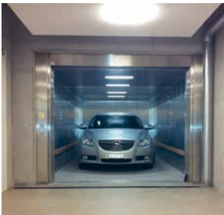
Underground car park - Zürich, Switzerland
